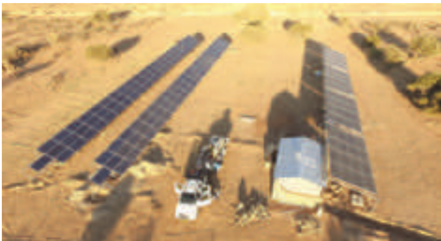
Figure 5: Installation of Project S-PV 1
