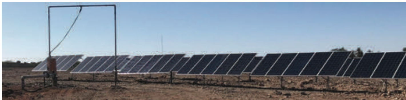
Figure 6.2: Installation of Project S-PV 2
