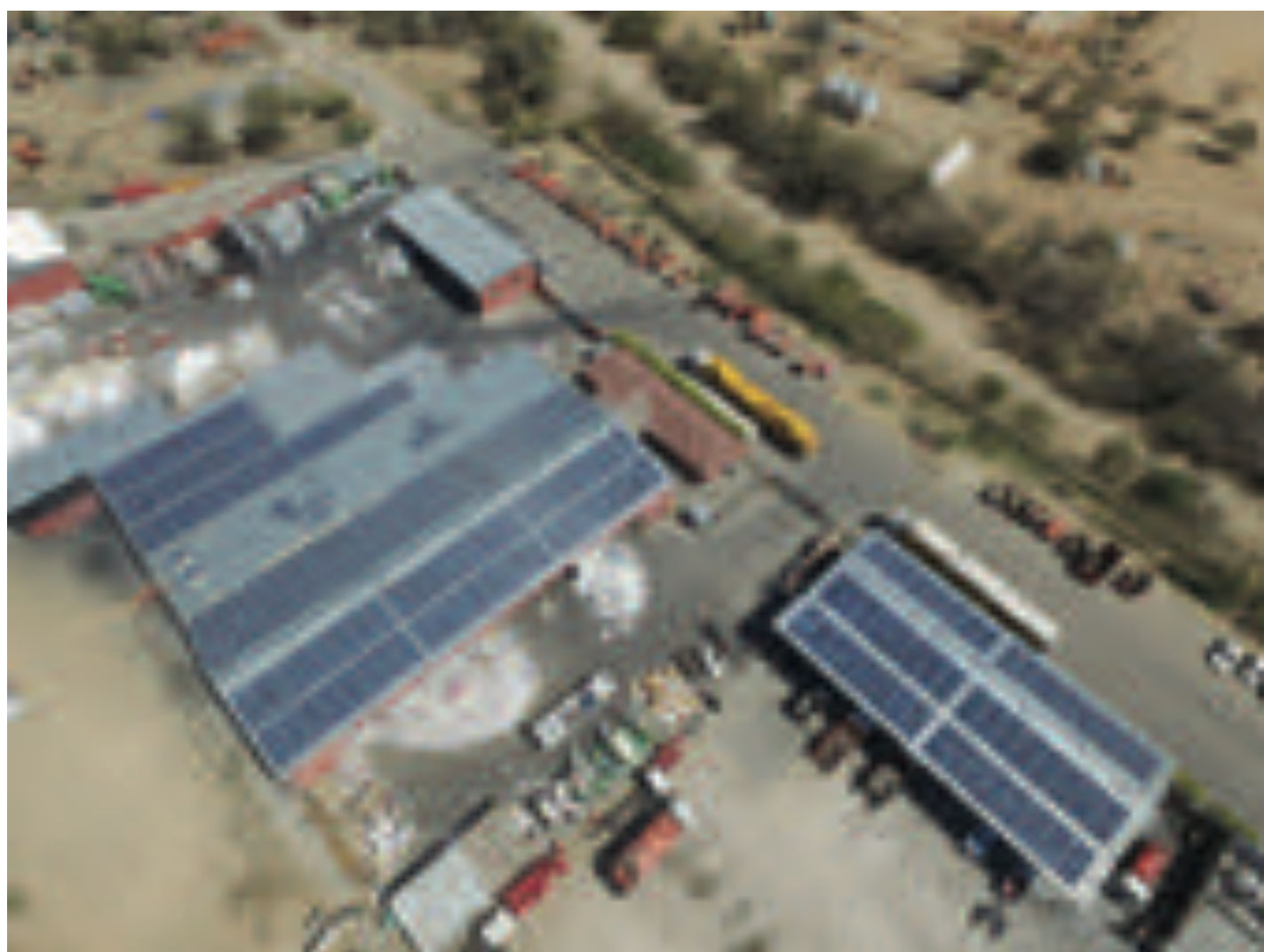
Figure 9: Installation of Project S-PV 5
