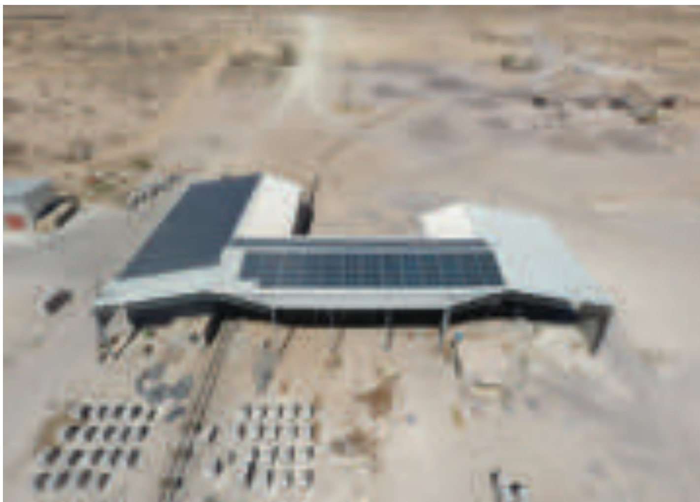
Figure 8: Installation of Project S-PV 4 (Mariental)
