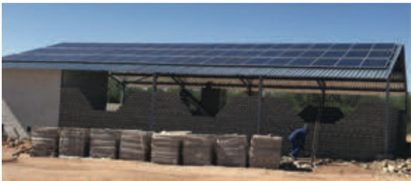
Figure 6.1: Installation of Project S-PV 2
